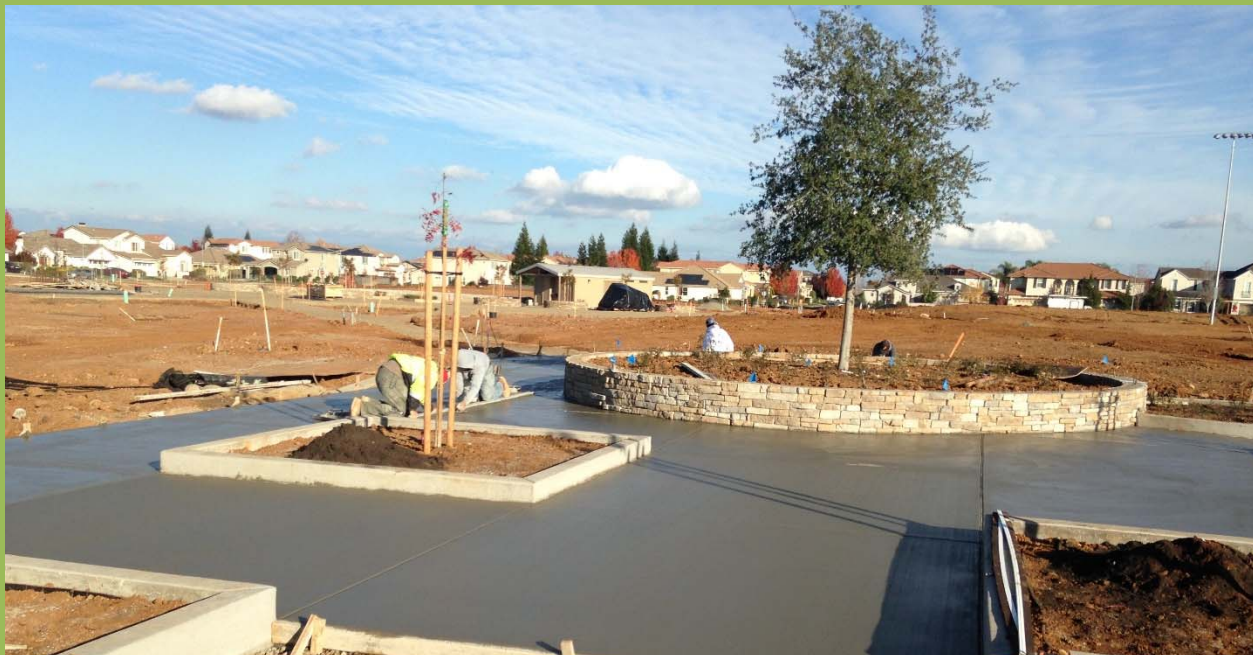
Seat Wall Construction and Landscaping Work Continues
