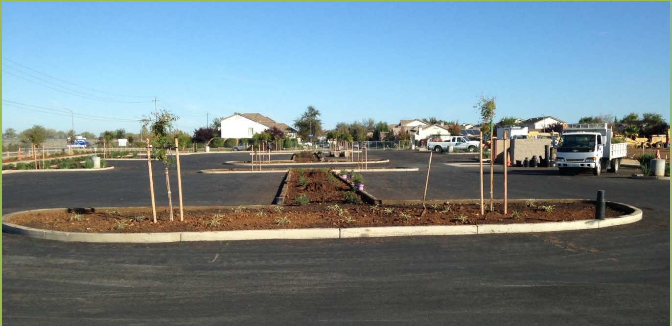
Parking Lot Paving Completed in November
