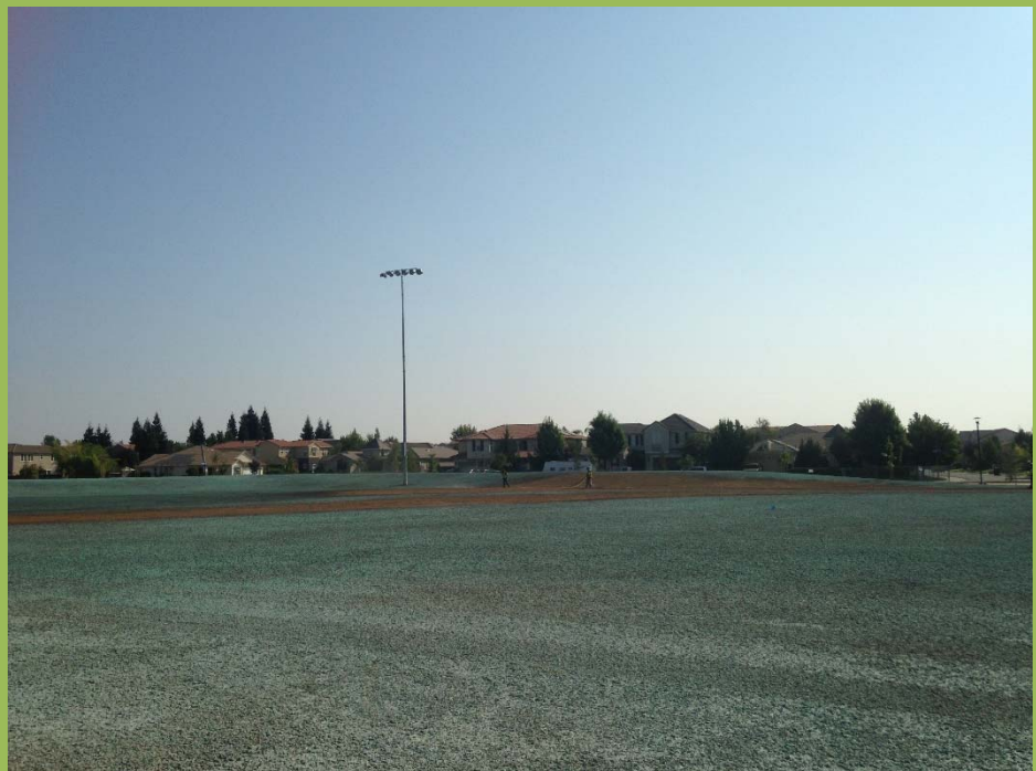
Hydroseed was applied in late September
