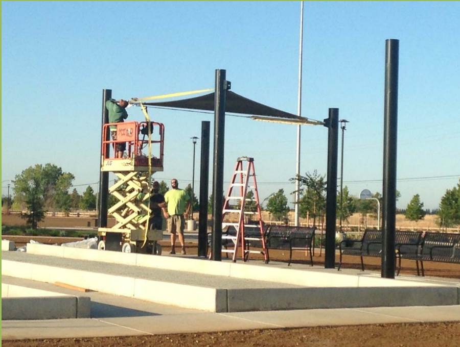
Fabric Canopies were installed in September
